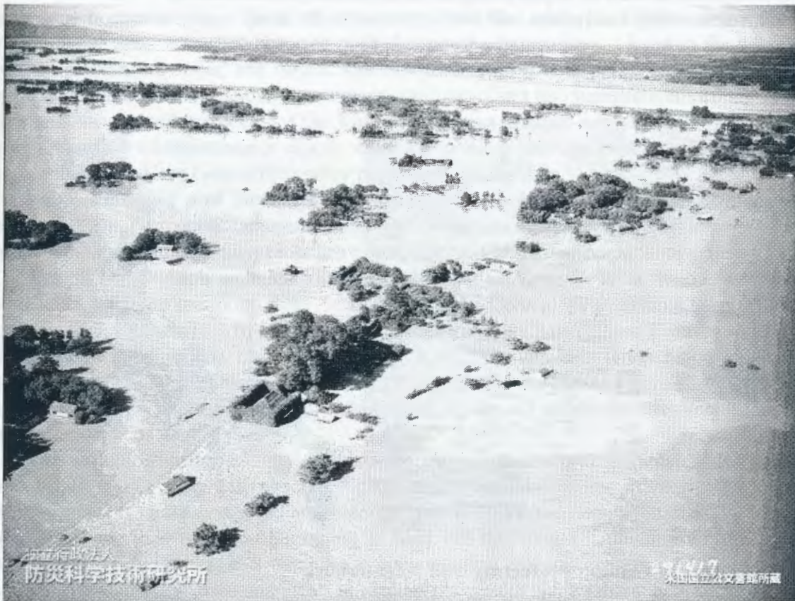
Fig. 1 Damage from Hurricane Kathleen, 1947
